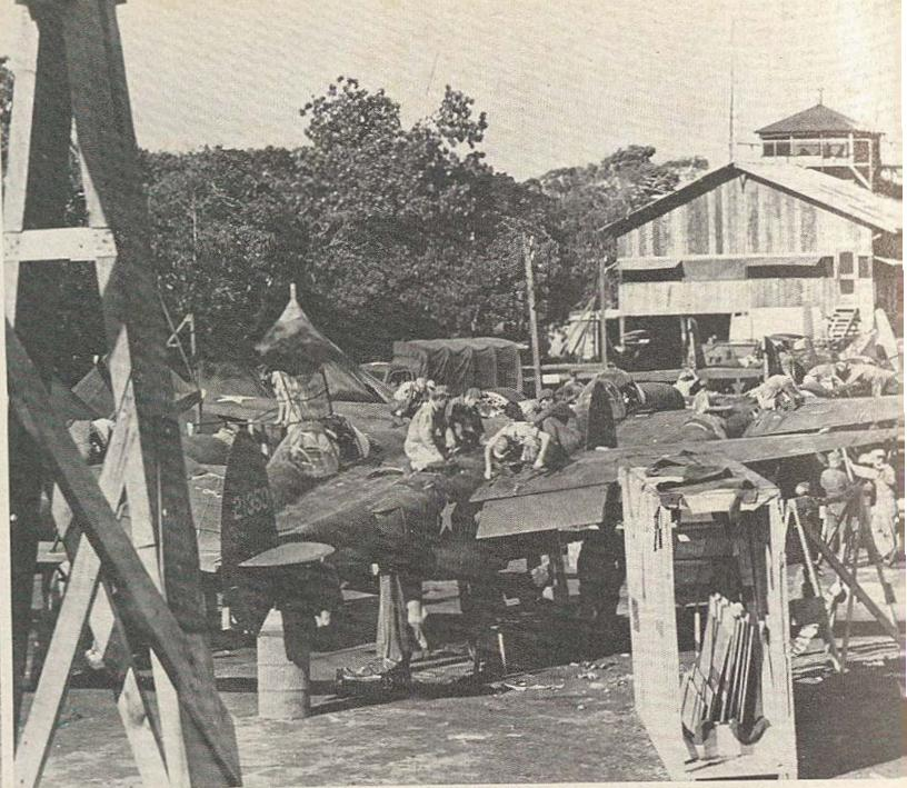
View of an assembly area of a South Pacific base where P-38 and P-39 fighter planes are put together.
