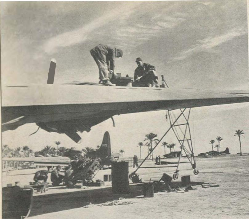
Repairing the damaged wing of a B-17 bomber in Middle East.
