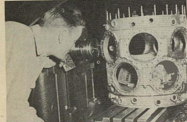
A precision machinist in the engineering shops matches crankcase sections for a 1200 horsepower aircraft engine.
