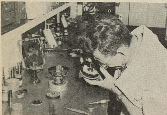
Overhauling a gyroscopic directional indicator is precision work.
