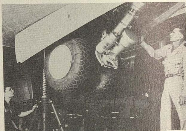
Checking landing gear on a B-29. A routine job at the world's largest depot at Kelly Field.
