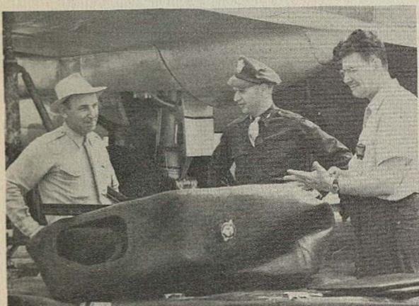
Rubber tanks are removed for inspection and repair while planes are going through overhaul.
