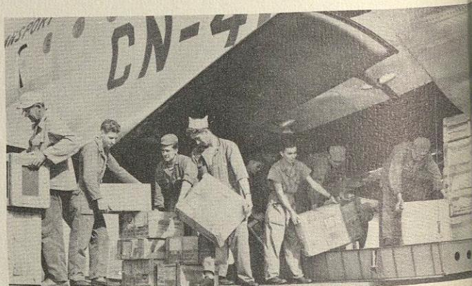
With a flat-bed truck positioned under the electric cargo elevator, men of the Cargo Warehouse, load equipment, which will be hoisted into fuselage.
