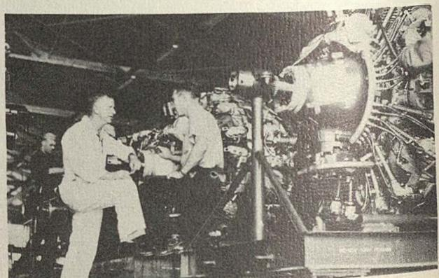
Mounting engines for airplanes going through overhaul.
