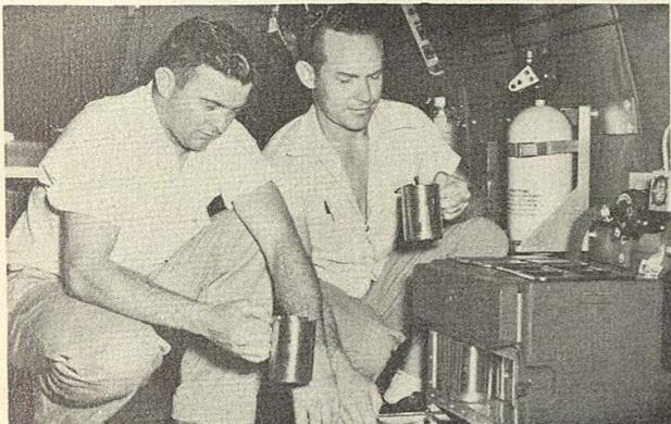
The very latest in air comfort is examined by L. A. Rogers (left) and Willard Lang. Electric food heaters were installed in fifteen B-29s at Kelly Field for operation in the cold weather regions of Alaska.
