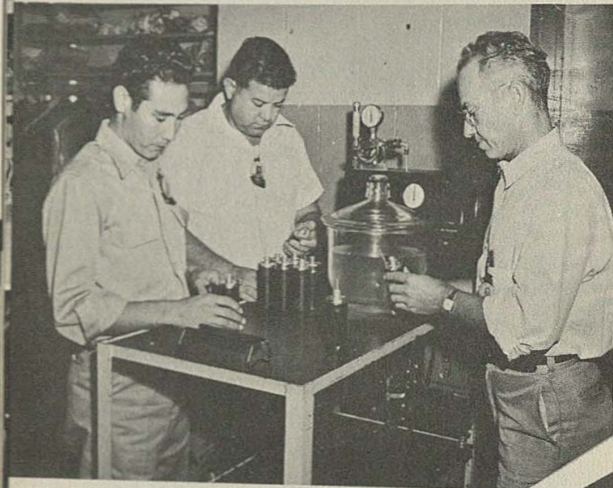
▼ Bldg. 320. Evacuating and hermetically sealing tachometer indicators.
