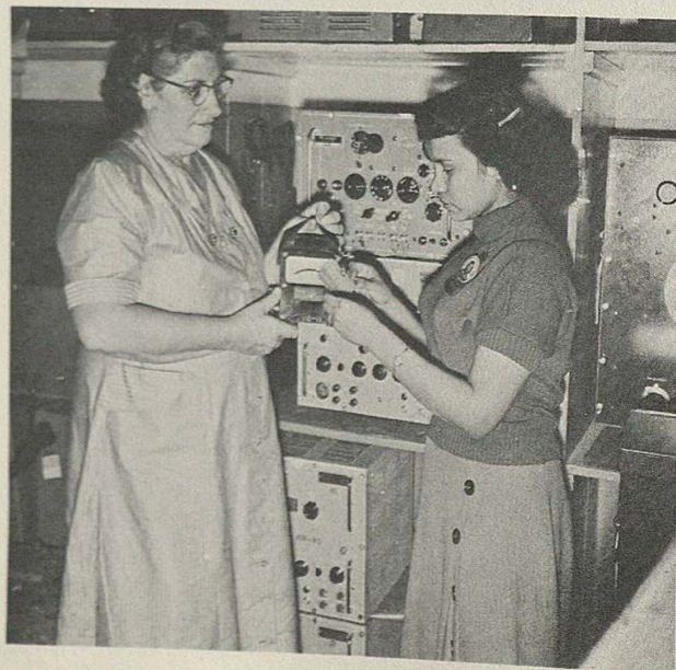
➤ Electrical meter being tagged for calibration recheck.
