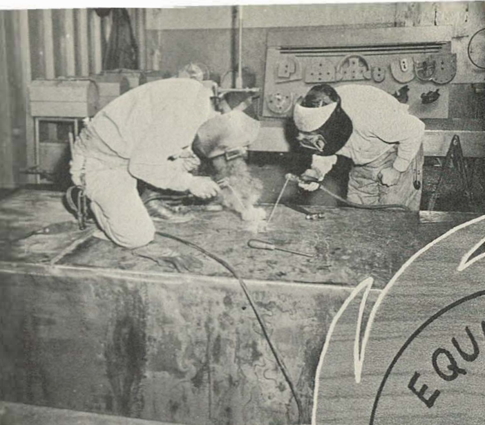
▲ Electric welding on storage tank section.
