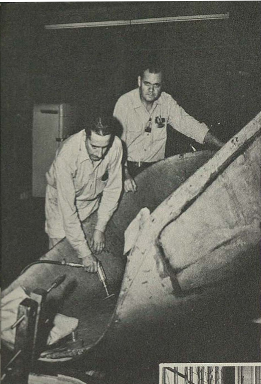
► Repairing a radome from a B-50 Aircraft under supervision of Mr. James Moak, right, Unit Chief, Glass Section. Bldg. 324.
