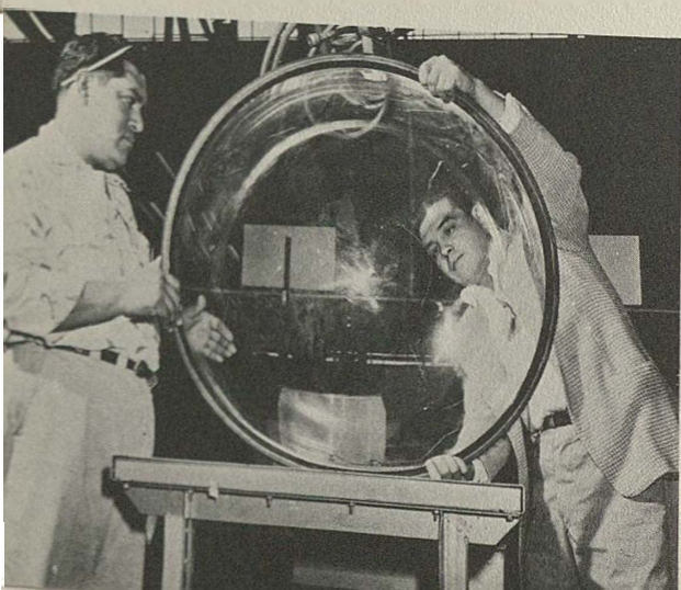
Mr. L. Salazar and Mr. Max Martinez of Glass Section inspecting a B-36 sighting dome. Bldg. 324. ►
