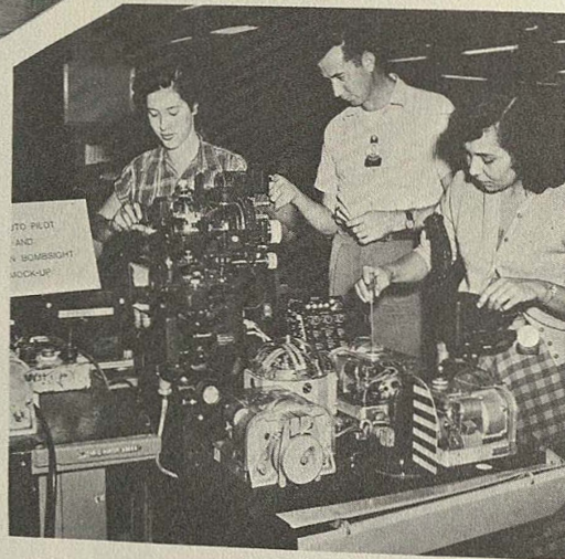
▼ Bldg. 326, adjusting C-1 auto pilots.
