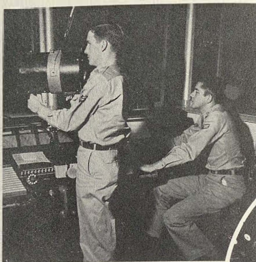
Above: Control tower operators directing traffic with light gun. Assistant relays messages to operations.
