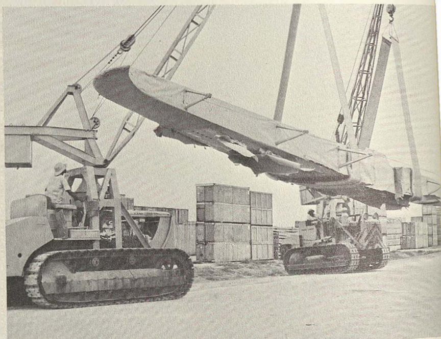
Mobile cranes handle the B-36 stabilizer with ease.
