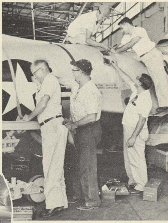
T-33 tail section disassembly
