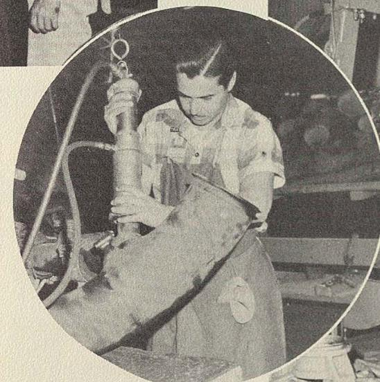
Tearing down an exhaust stack
